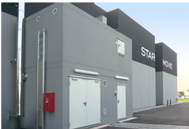
Double-floor heating module 200 kW wood chips, business
